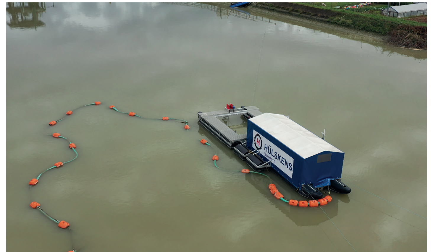
FIGURE 4 SediMover-130 at a project in Italy during continuous sediment transfer.
