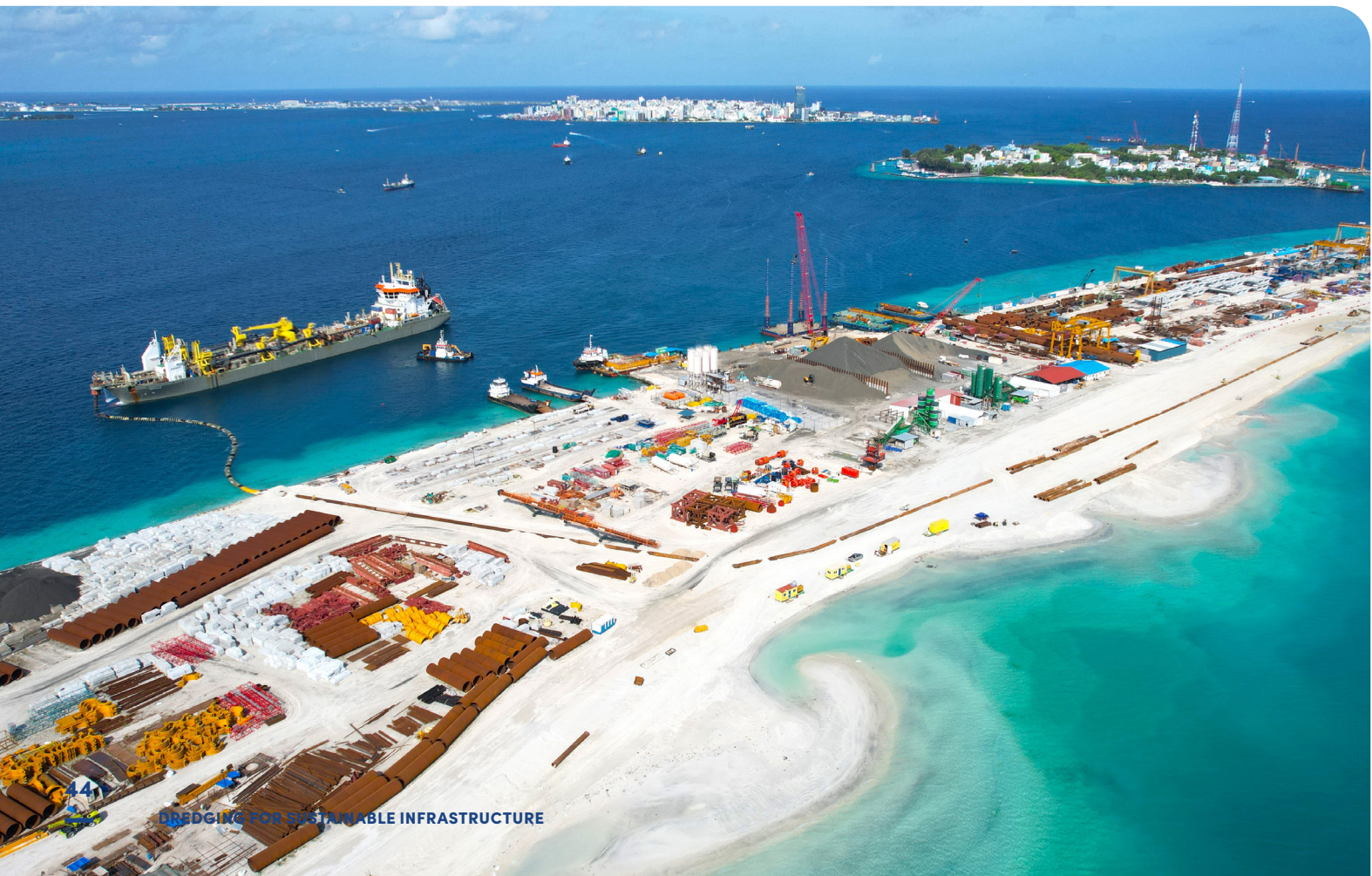
The trailing suction hopper dredger Oranje pumps sand to the reclamation area.
