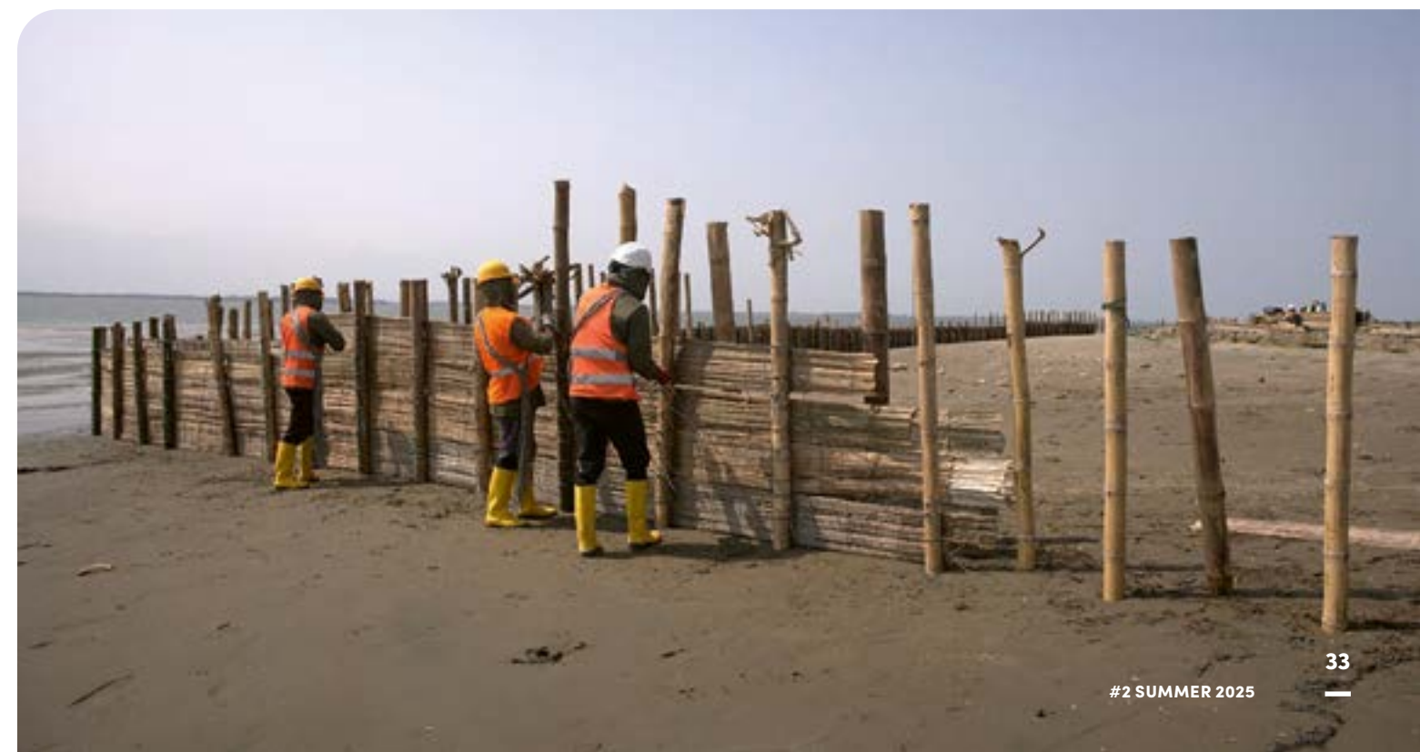
Fishermen from the partner associations building the locally designed, semi-permeable structure using natural materials.
