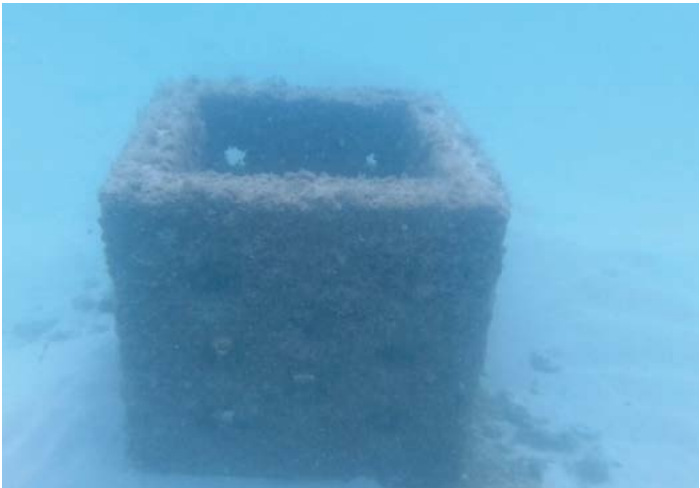
FIGURE 4 Type D fish domes: concrete boxes.
