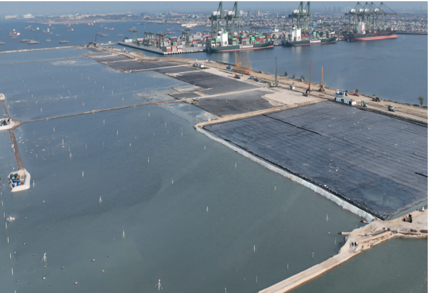
FIGURE 5 Kalibaru project. Construction of new land for the Kalibaru terminal in the port of Tanjung Priok, Jakarta, Indonesia.
