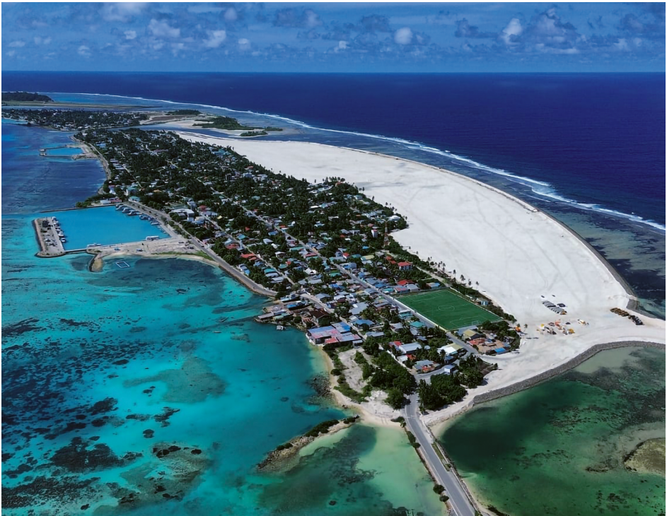
FIGURE 18 Maradhoo reclamation footprint on 14 August 2023 (drone photo taken from the north edge of the reclamation). The location on the north side where the floating pipeline cross the main street is indicated with red box.
