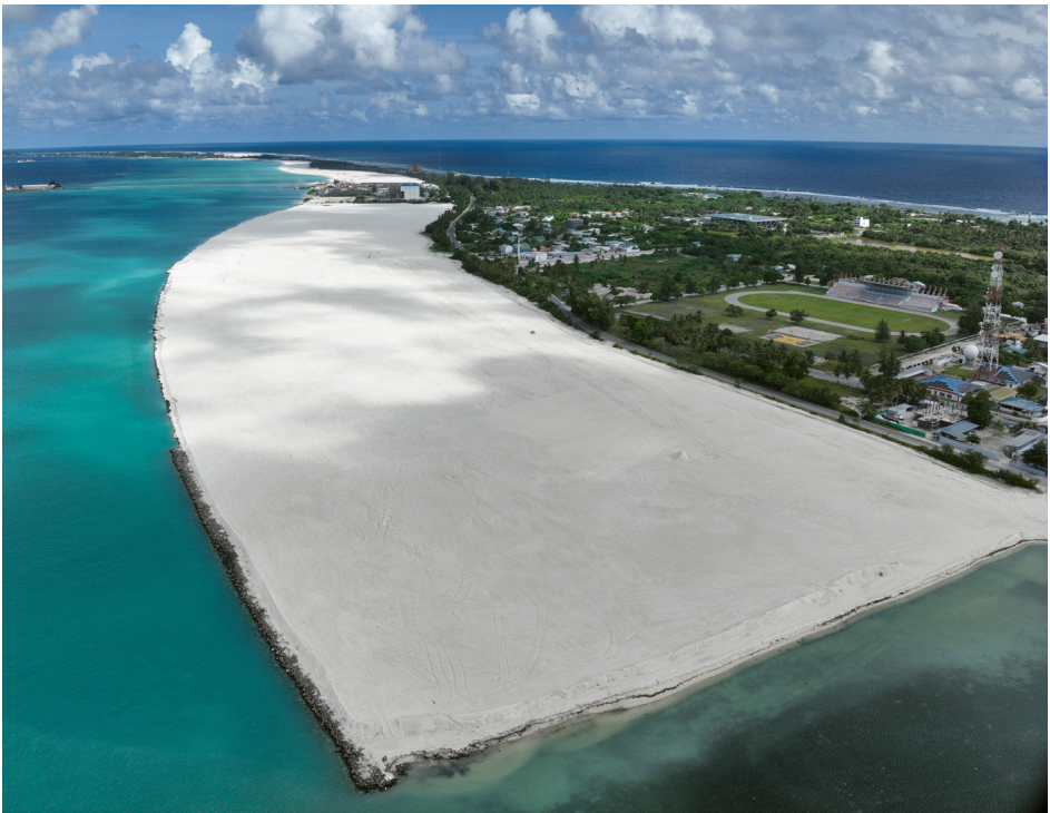
FIGURE 19 Hithadhoo zone 1 reclamation on 13 August 2023 (drone photo taken from the north side of the reclamation).
