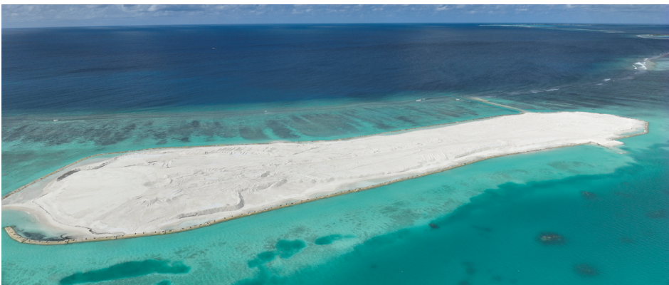
FIGURE 21 Resort island 2 reclamation on 13 August 2023 (drone photo taken from the south of the island). The opening used as reclamation exit is visible in the west of the island.
