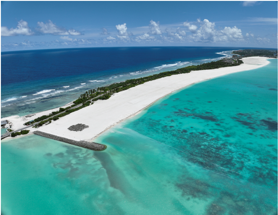
FIGURE 16 Reclamation at Hithadhoo zone 2 on 14 August 2023, with groyne constructed in the south of the reclamation and the natural beach started forming in the inner side of the atoll.
