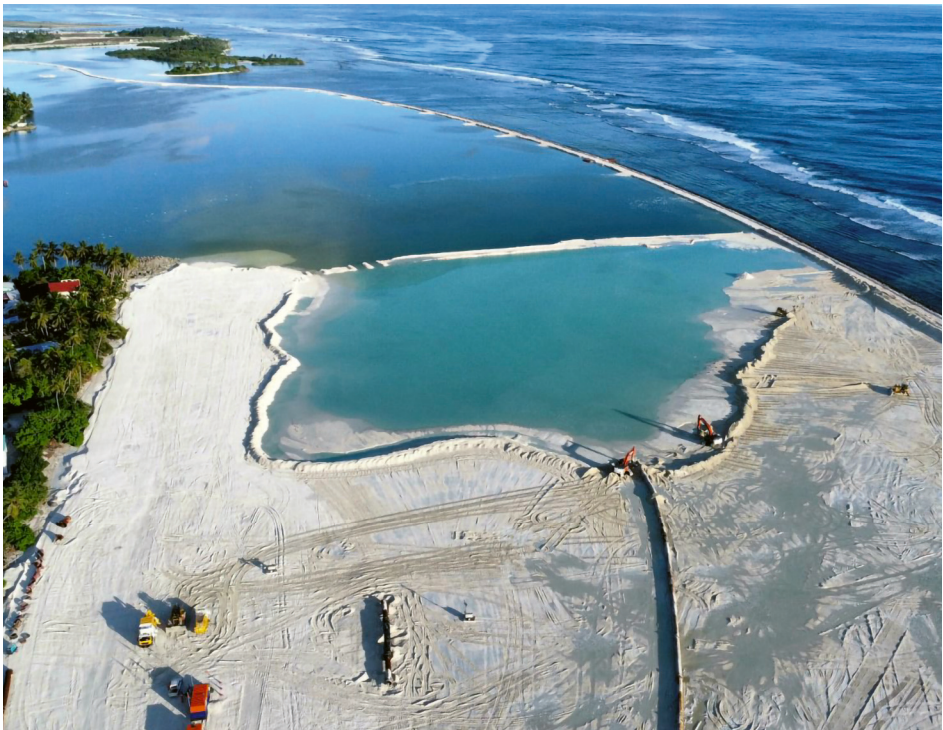
FIGURE 17 Maradhoo reclamation footprint progress on 12 June 2023 (floating pipeline discharging sediment mixture from the north).
