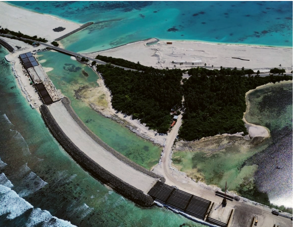
FIGURE 23 Hankedere reclamation completed on 14 August 2023.
