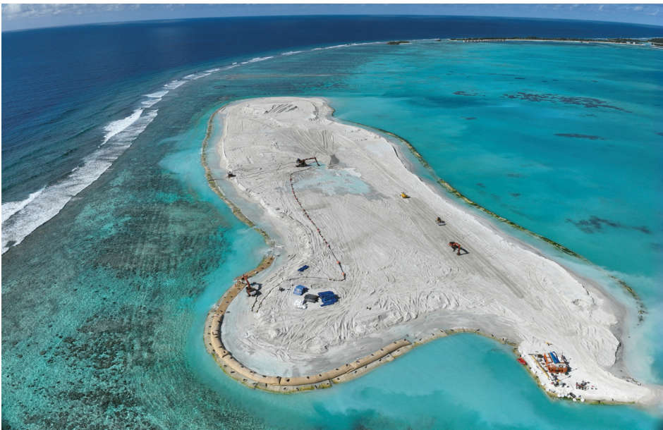
FIGURE 22 Resort island 3 reclamation footprint on 14 August 2023 (drone photo taken from the west of the island). In the lower left of the photo you can see the second layer of geotextile tubes being installed.
