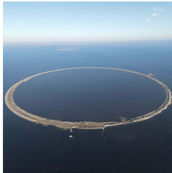
FIGURE 20 New donut-shaped soil depot on the southern island.
