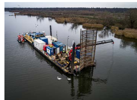
FIGURE 15 Executing the clearance works in the fairway.
