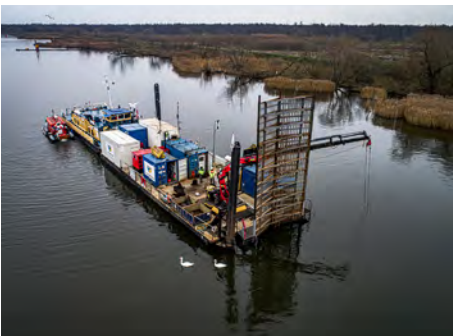
FIGURE 15 Executing the clearance works in the fairway.
