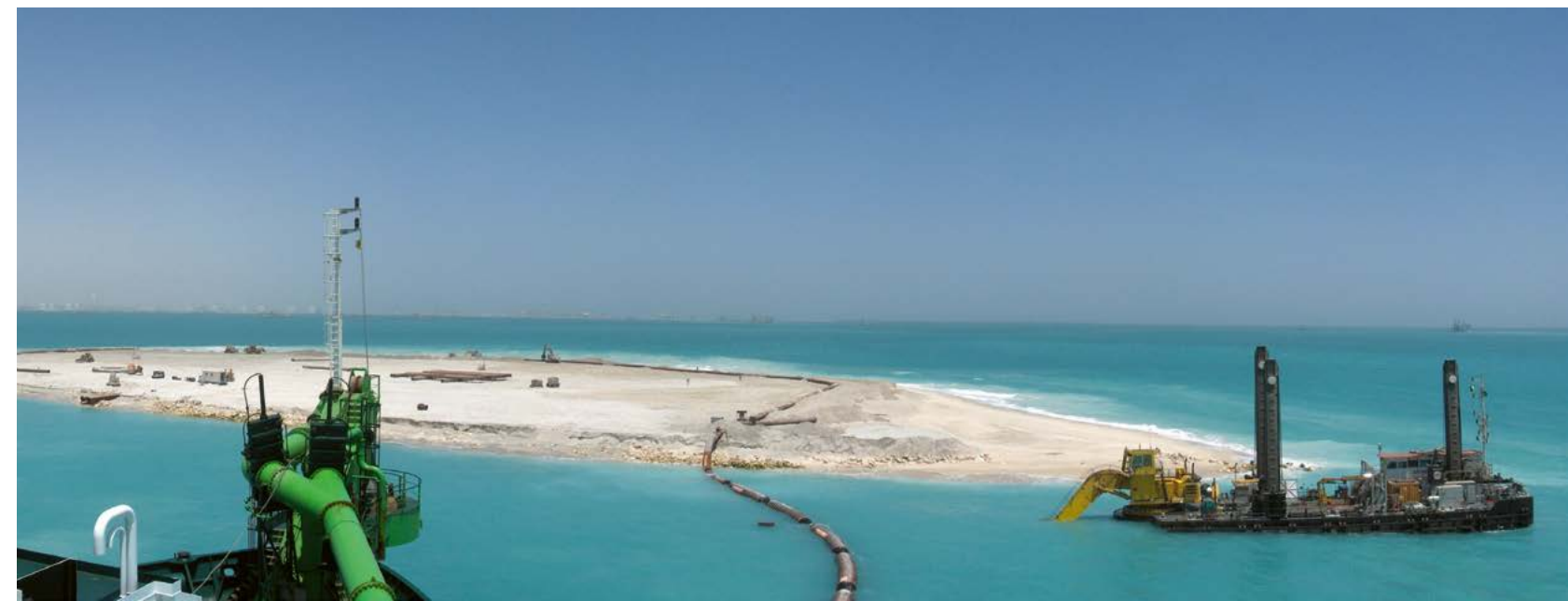
FIGURE 4 Pricing of marine equipment using CIRIA tables provides benchmark rates.
