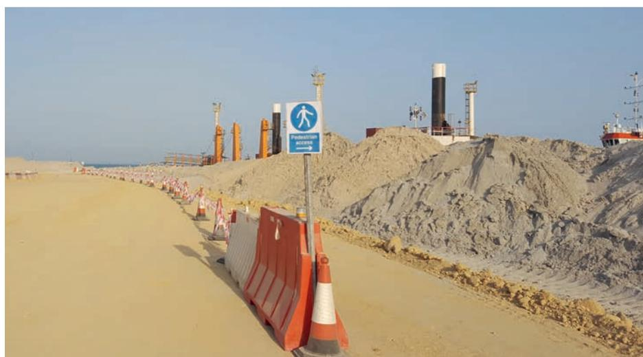
Figure 2: Clear signage (must be lighted in the dark) should be utilised to indicate pedestrian walkway to prevent any incidents with moving vehicles.
