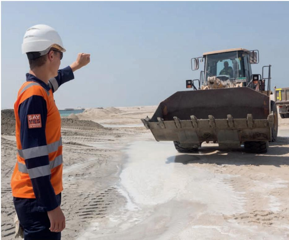
Figure 1: A banksman directing a moving vehicle on the construction site.
