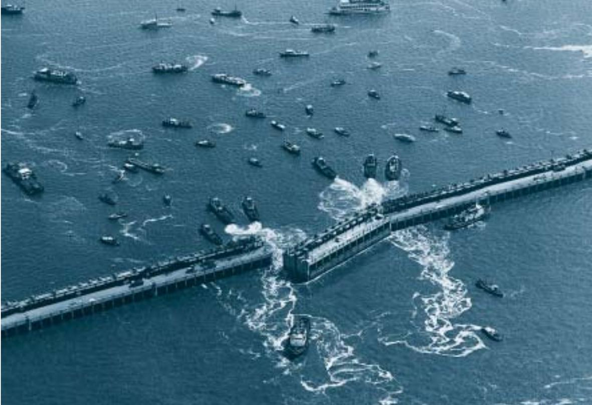
Figure 9. One of the spin-offs of the Delta Project: discharge caissons at the Oosterschelde, being built in 1976.
