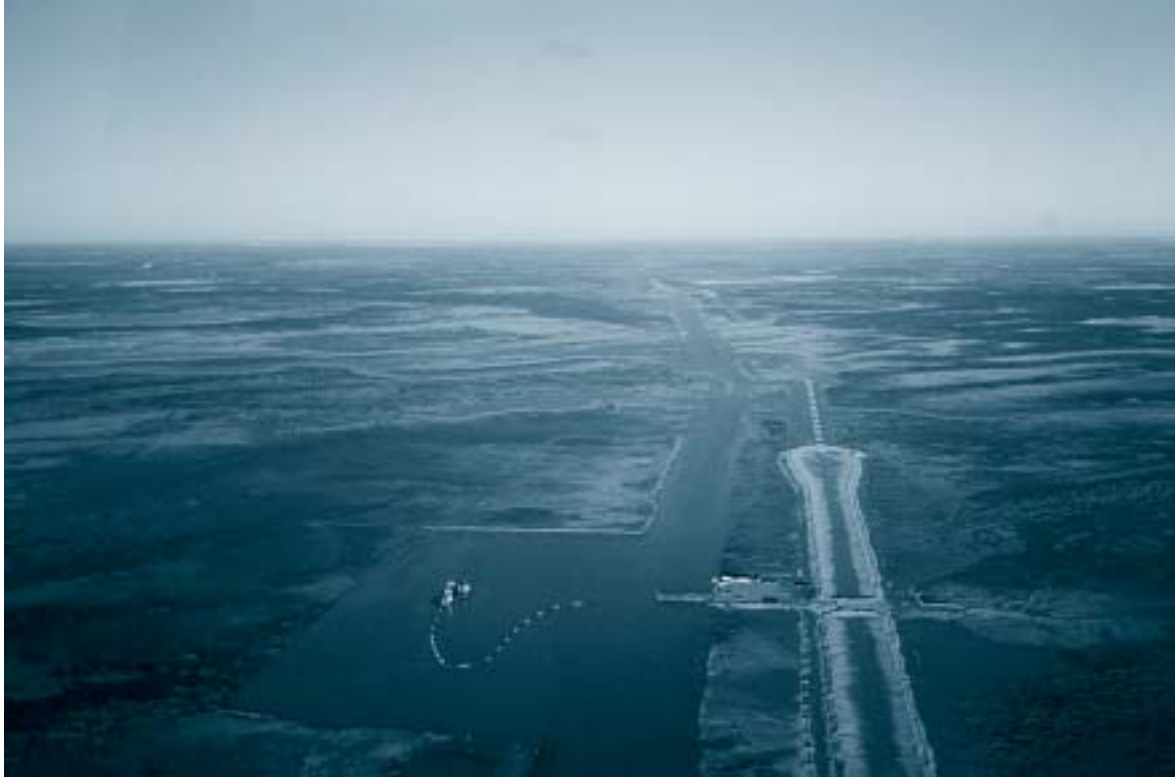
Figure 5. Cutter suction dredger Zuiderklip dredging sand in a borrow pit and filling an intermediate layer of an embankment – view from Victoria (East) with respect to the Connection.
