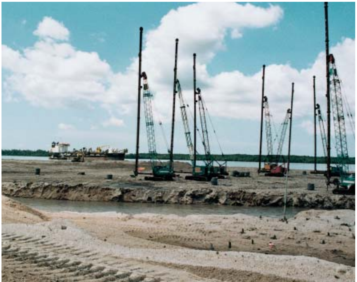
Figure 10. Some 20 million metres of vertical drainage (wick drains) were installed.
