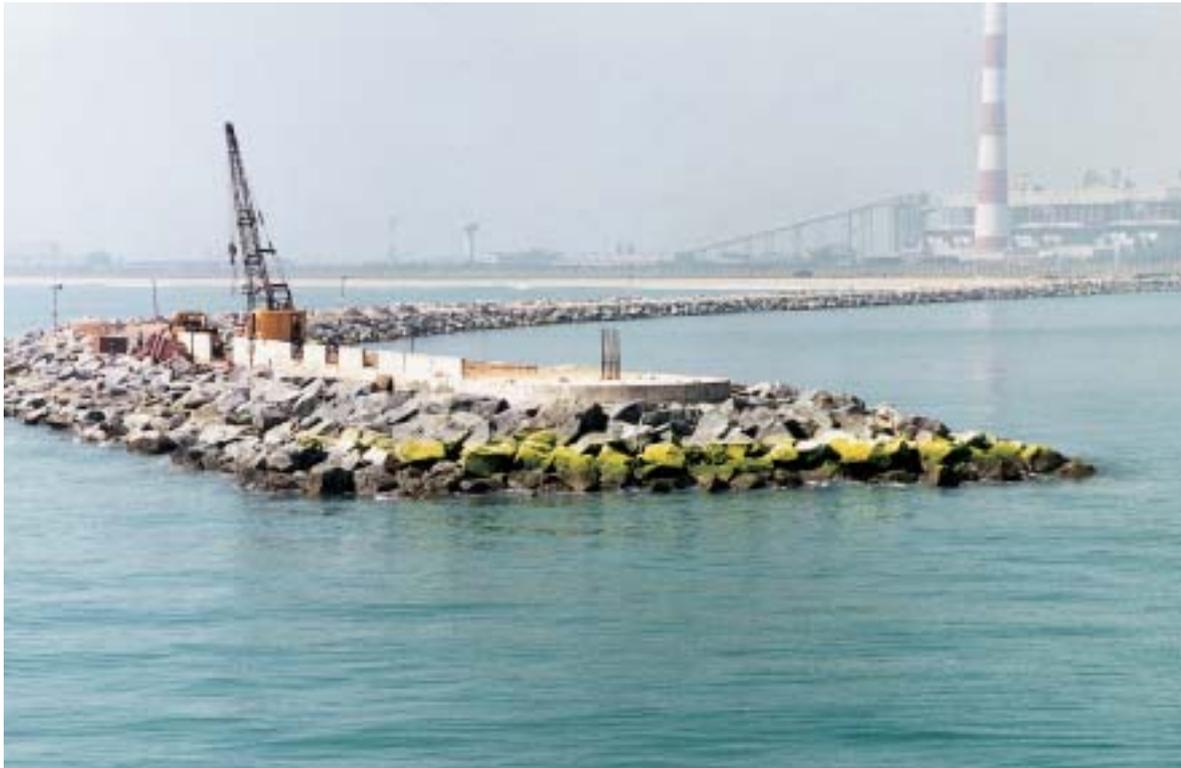
Figure 7. The placing of in situ concrete slab and wave wall at the South Breakwater under construction.
