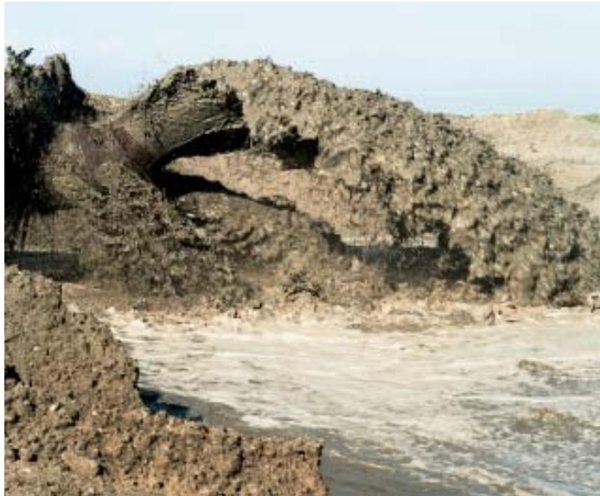
Figure 3. On-land discharge of the dredged materials.
