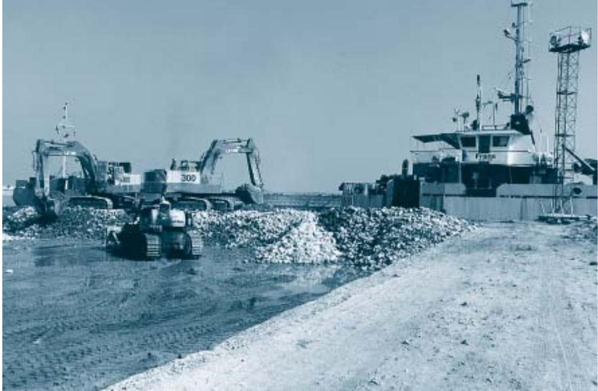
Figure 3. The side stone dumping vessel Frans being loaded at the temporary work harbour.
