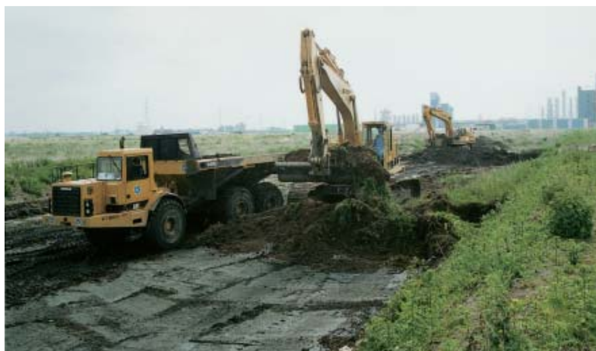
Figure 1. At Kallo in Belgium, dewatered and treated silt is being placed at a test site.
