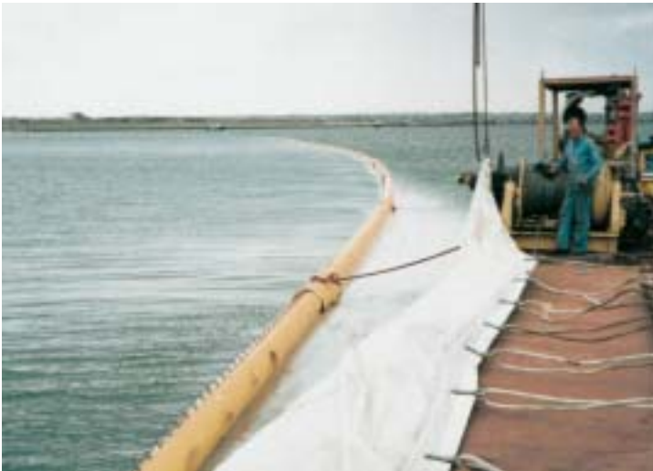
Figure 4. The floating silt curtain anchored to the bottom kept suspended solids (bottom materials disturbed by dredging) from spreading throughout the bay.
