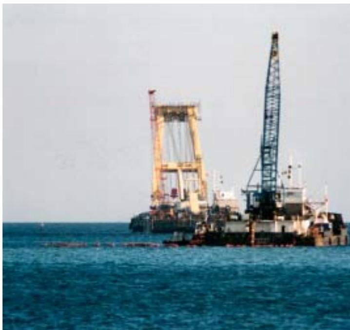
Figure 4. After backfilling, the area was compacted using twin torpedo vibro-compactors supported from the crane barge *Kutxa*. *Kutxa* is seen here dredging under the gas line, with a pull barge behind.
