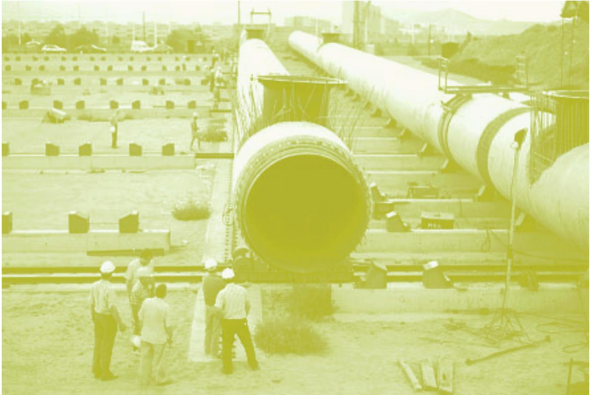
Figure 2. The first pipe string being moved from the welding area to the stock area. The structures on top of the pipe are the starters for the diffusers.
