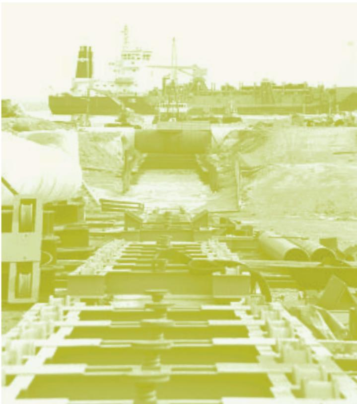
Figure 3. Cutter dredger Rozenburg, 160 m from cofferdam and hopper dredger Lelystad, 600 m from cofferdam, launching preparations on shore side.
