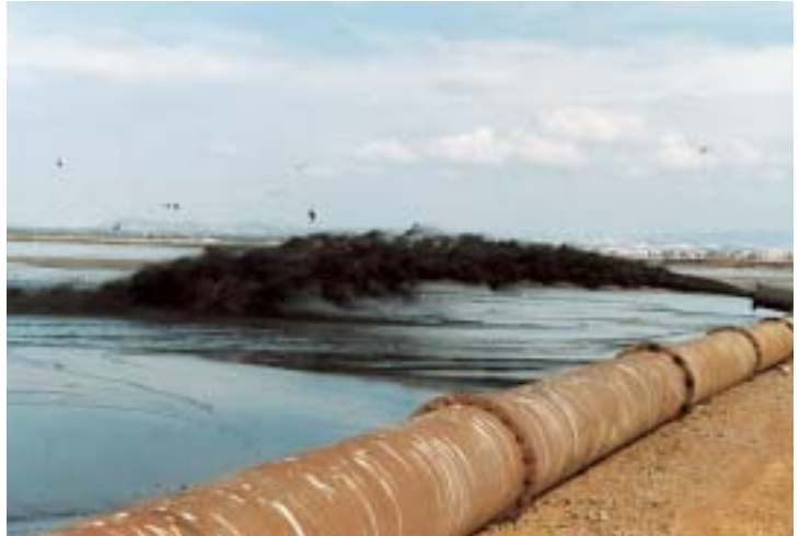
Figure 4. Millions of cubic metres of mud, sand, gravel and shells were pumped sometimes as far as 6,000 metres.
