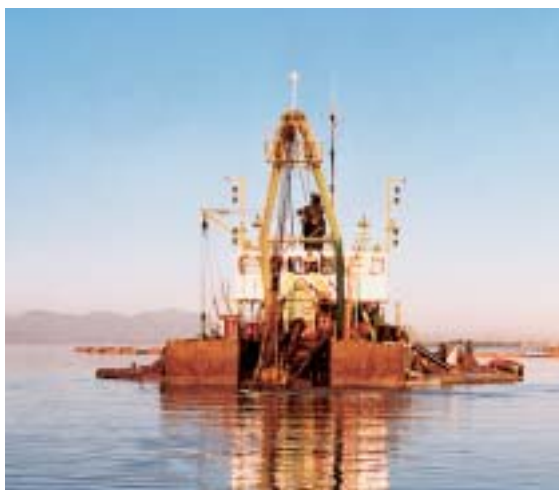
Figure 3. One of the two cutter suction dredgers which were modified in order to be able to dredge in the very shallow waters of the lagoon.
