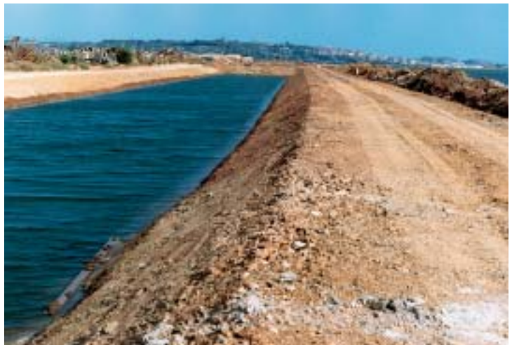
Figure 5. The drainage canal which was constructed to collect the water of the Rio Sestu and carry the urban and industrial waste away from the lagoon.
