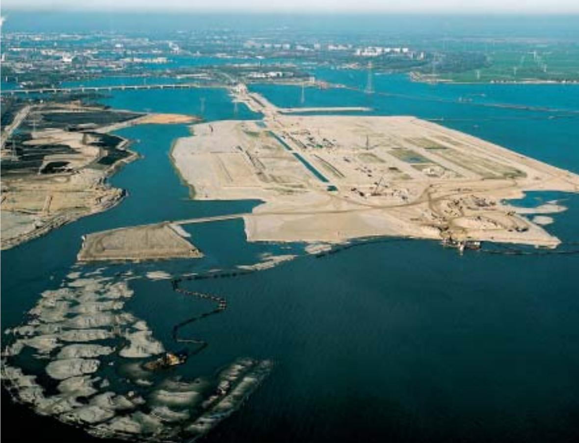
Figure 20. The construction of “sand pancakes” by a spraying pontoon. The first sand layer was typically not more than 50 centimetres. The following layers have a thickness of between 0.6-0.8 metres.
