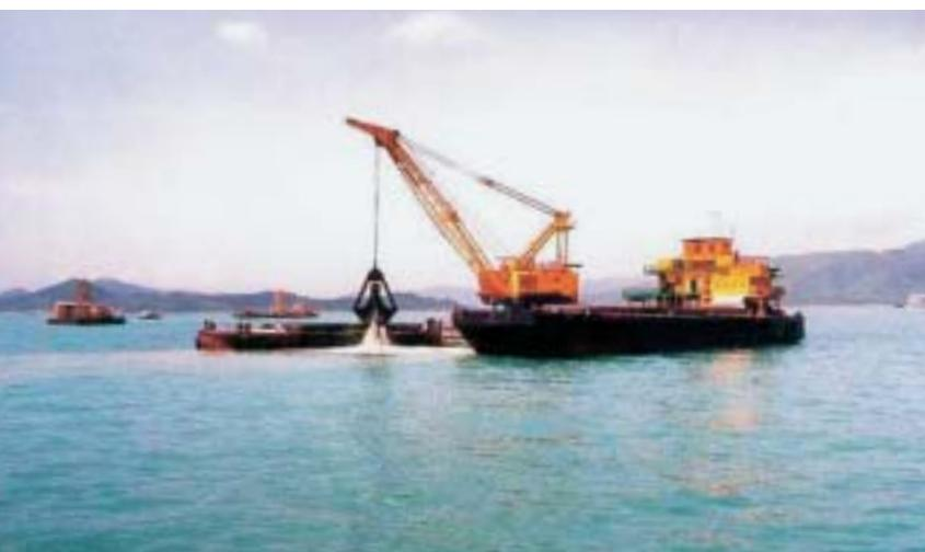
A solid foundation for the reclamation was found at levels varying from -10 m PD to -39 m PD, in some spots even -45 m PD. This meant that a mud layer of up to 33 metres thick was to be removed prior to the actual reclamation works.
