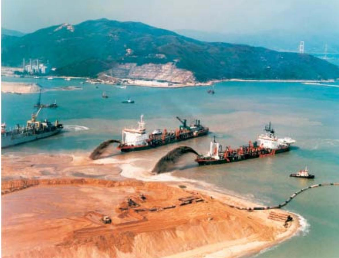
Figure 4. Large trailing suction hoppers during sand placement.
