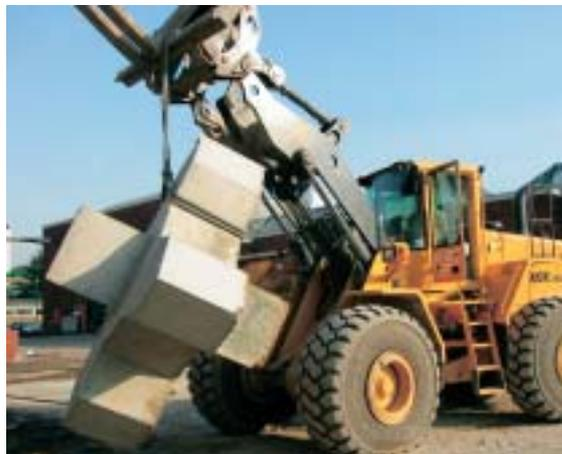
Figure 17. Handling the Xbloc® with a sling around the nose was the most suitable technique for placement.
