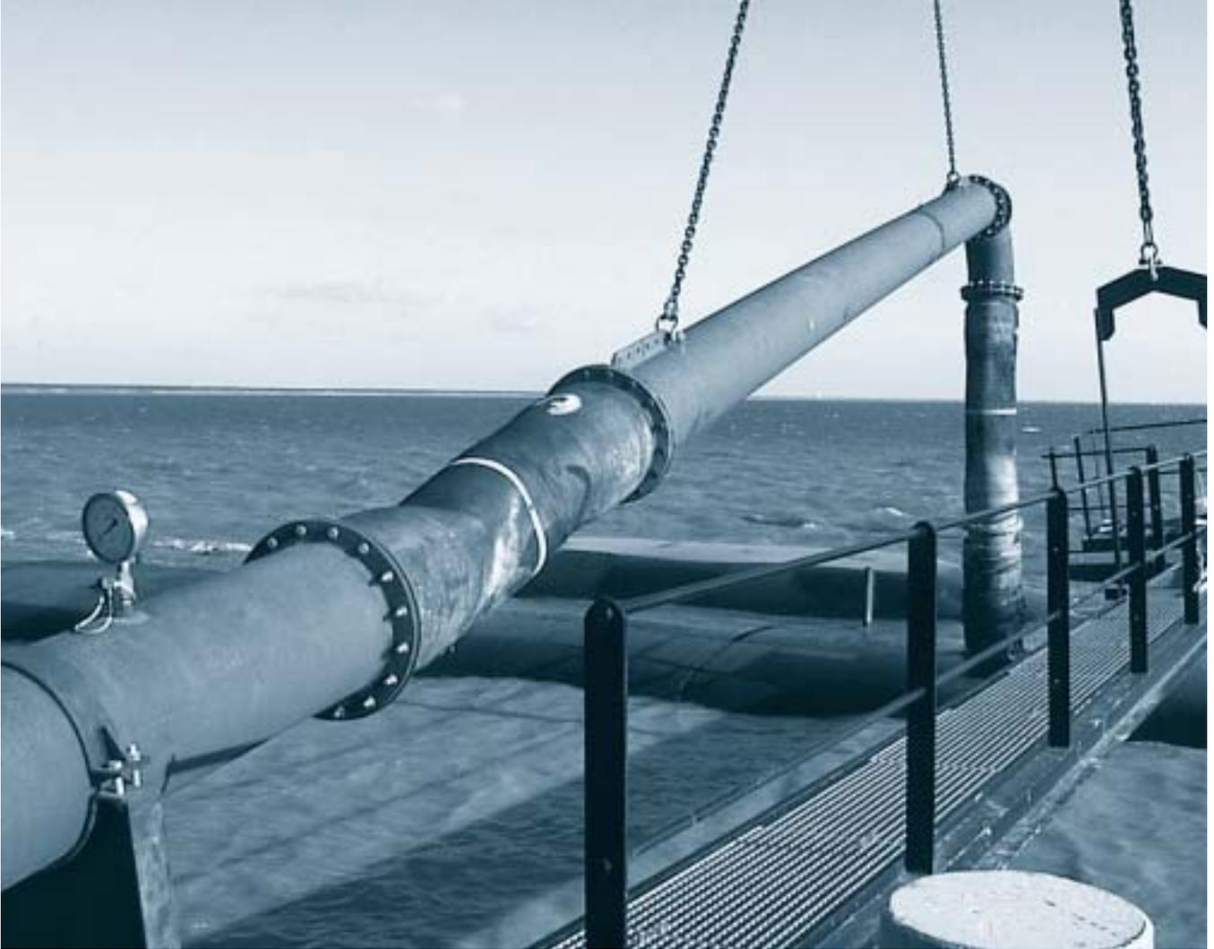
Figure 3. The connection point of the filling pipe and the geotube.
