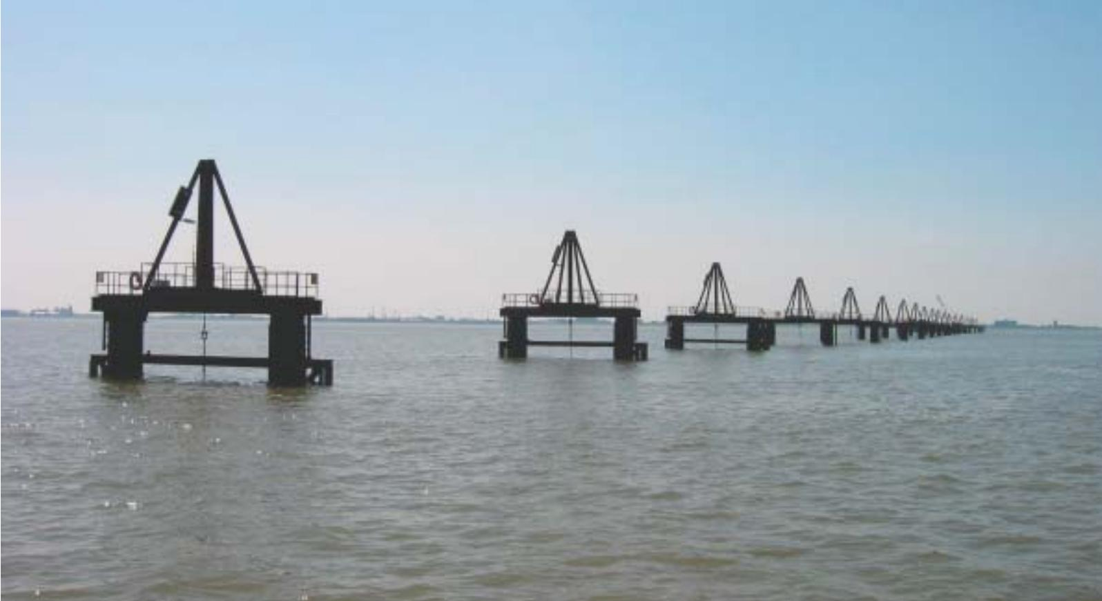
Figure 2. Support frames for holding the pipeline during dredging works as well as for during the lowering of the pipeline.
