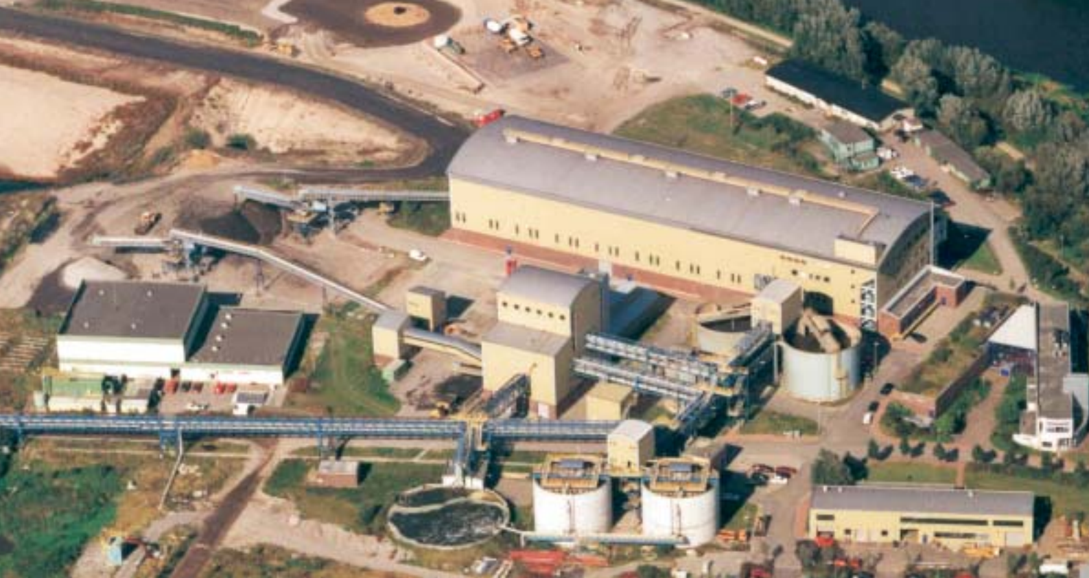
Figure 7. METHA plant – Mechanical treatment and dewatering of harbour sediments.
