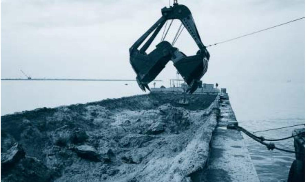
Figure 14. Loading of blasted rock into hopper barge.
