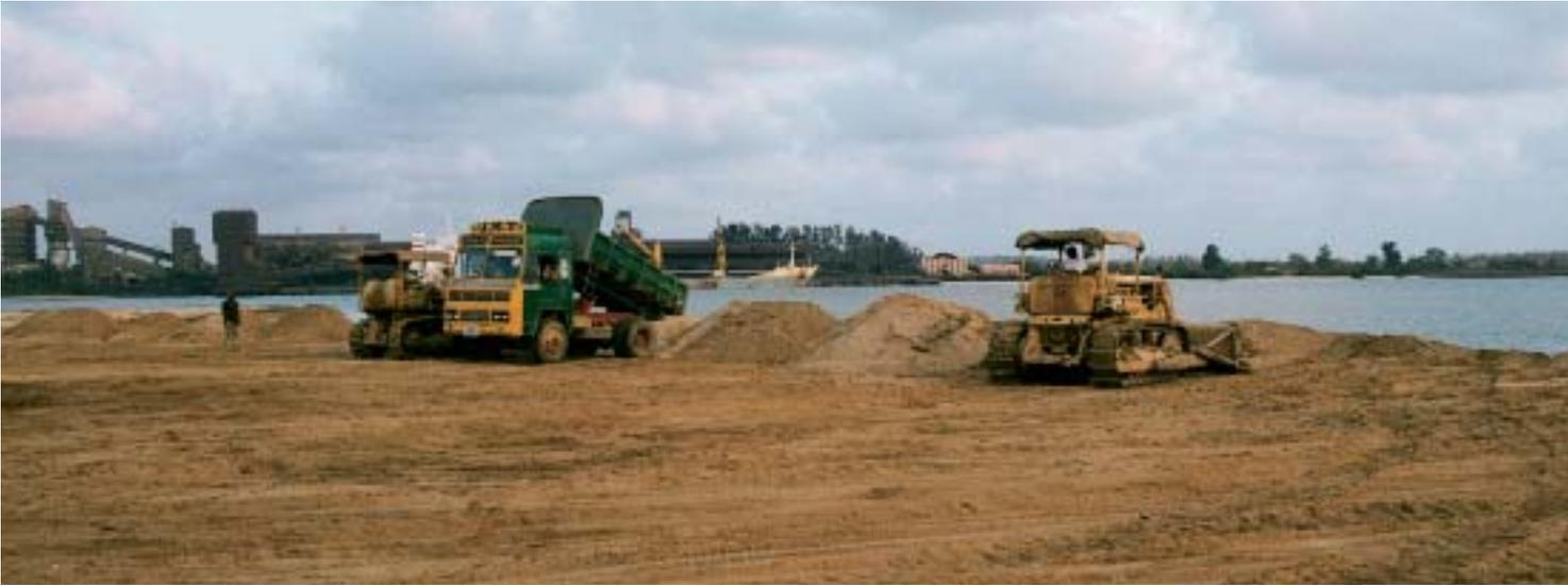
Figure 5. Dry excavation and disposal.
