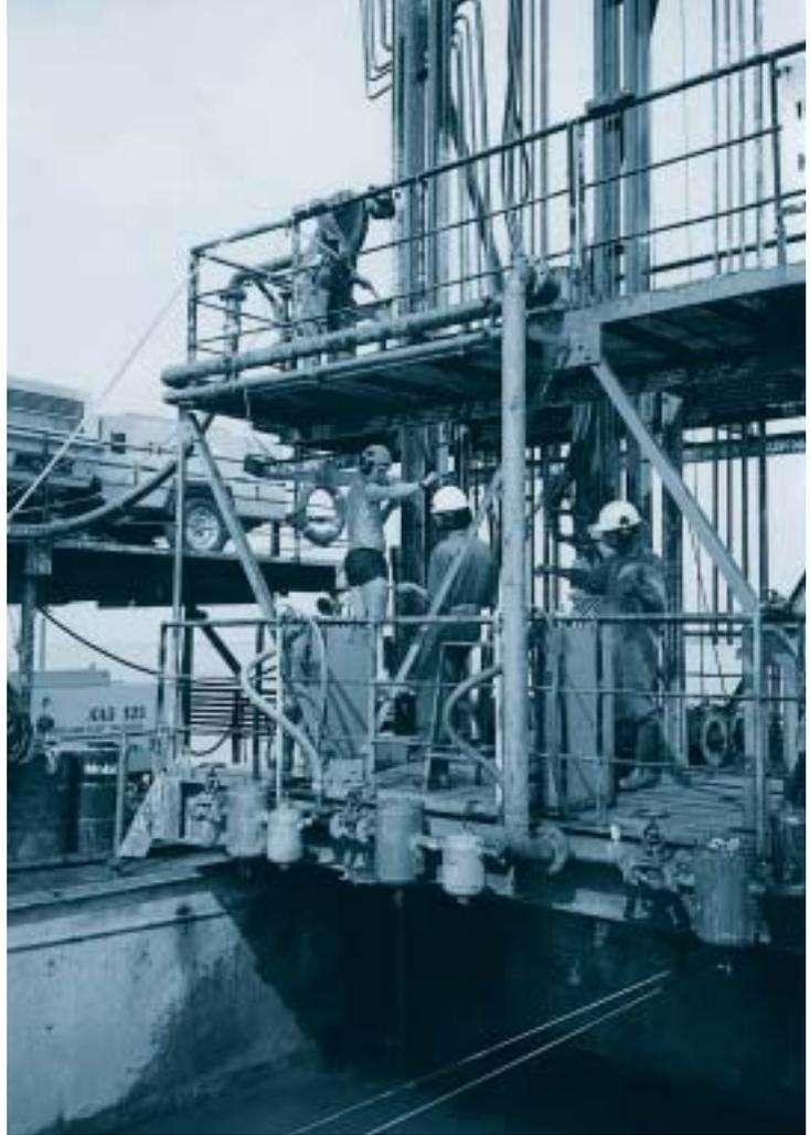
Figure 12. Overburden drilling in process.
