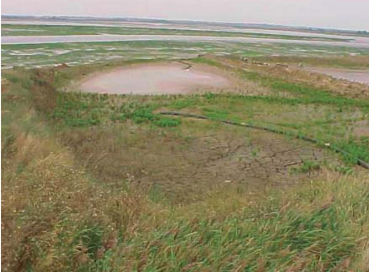
Figure 4. In 1998 and 1999 fine-grained dredged material was placed at Titchmarsh Marina in the UK to create mudflats and saltmarshes. Seen here, the placement stage.
