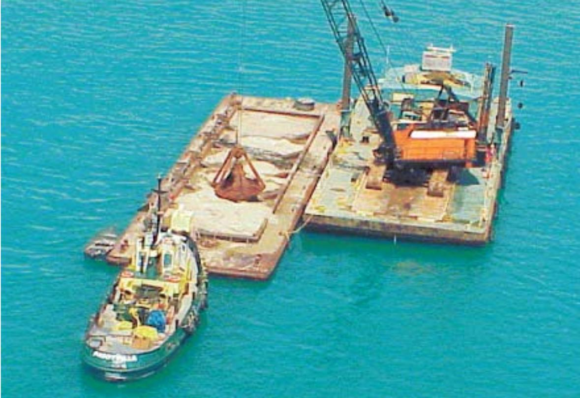
Figure 3. A clamshell dredge filling a dump scow in July 2002 in the South East Bend (SEB) Cut-Off Channel at the mouth of Lake St. Clair. This Channel is part of the main shipping and navigation route connecting all the Great Lakes.
