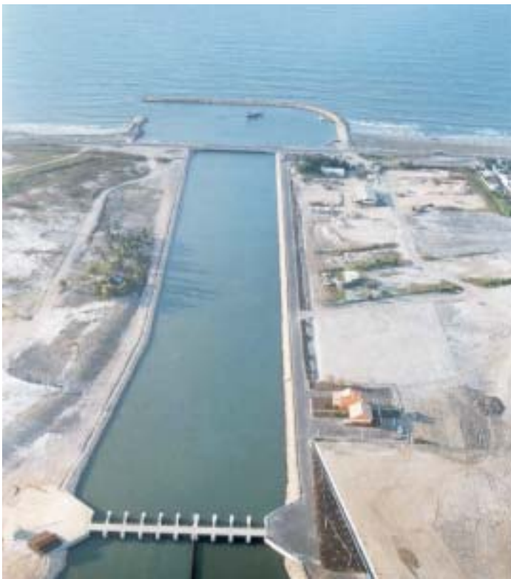
Figure 3. Photograph of the Tidal Inlet which has been placed near the pollution sources.
