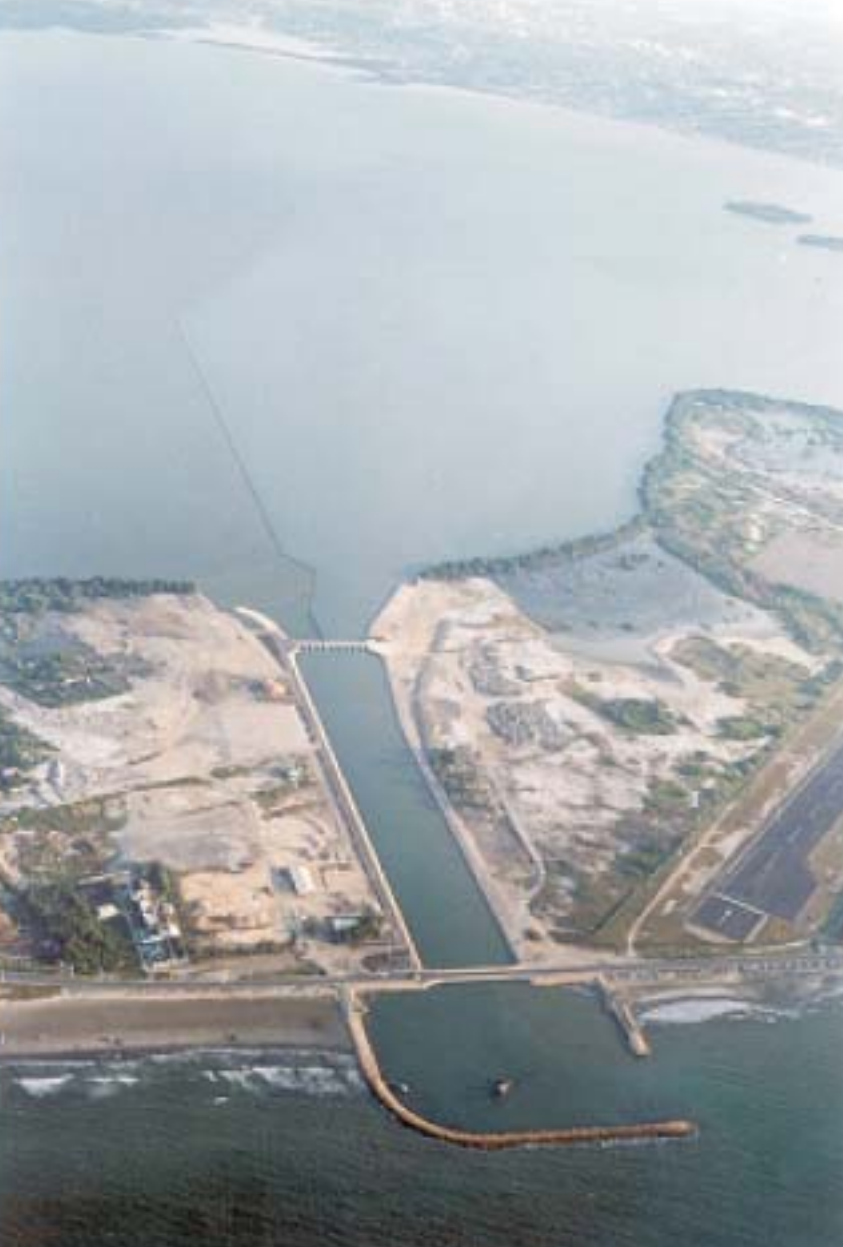
Figure 6. Aerial view of the channel, sluice complex and box-culvert.
