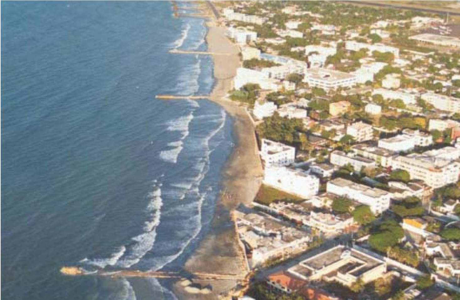
Figure 12. Under construction: Three new groynes were constructed and an existing one was extended.
