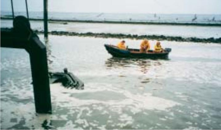
Figure 3. Turbidity measurements in progress with small vessels around the auger dredge during clean-up dredging in the Sea Harbour Channel, Delfzijl, The Netherlands.
