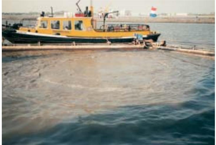
Figure 1. Turbidity caused by clamshell dredging contained within a siltscreen enclosure in the Geul Harbour, Port of Rotterdam.
