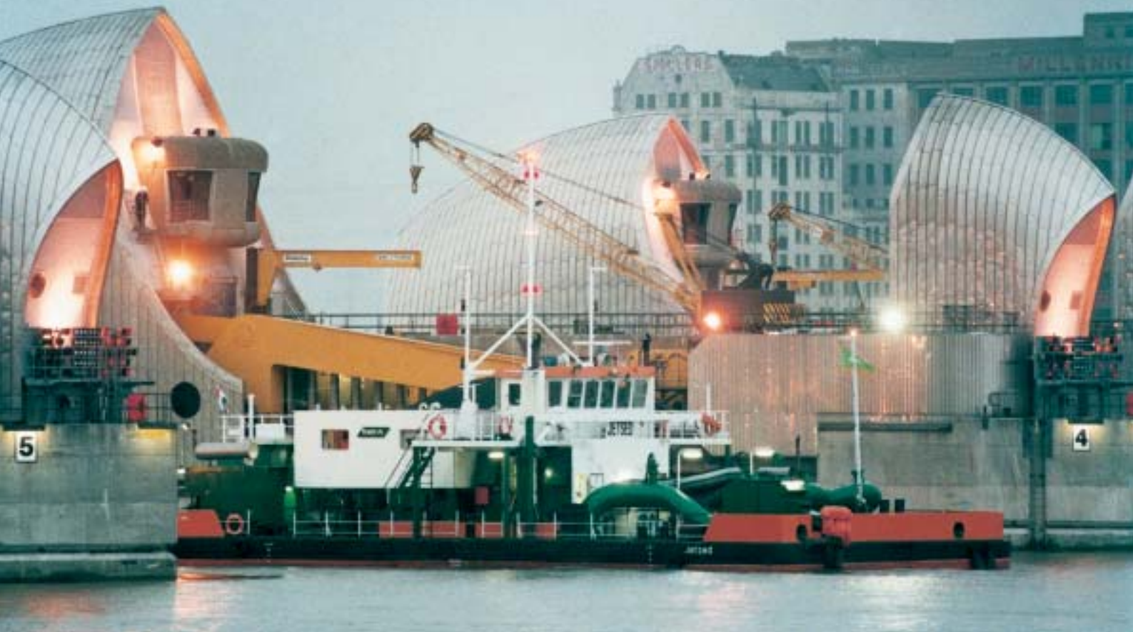
Figure 7. The water injection dredger Jetsed working close to the Thames Barrier Clearance.
