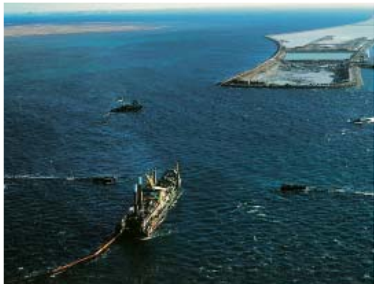
Figure 4. Cutter dredger Castor and gravity anchors in the Øresund (photo: Jan Kofod Winther).
