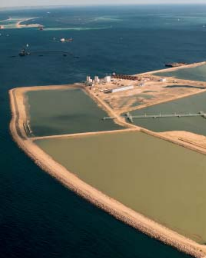
Figure 2. Progress of the works at 12 July 1996 (photo: Jan Kofod Winther).
