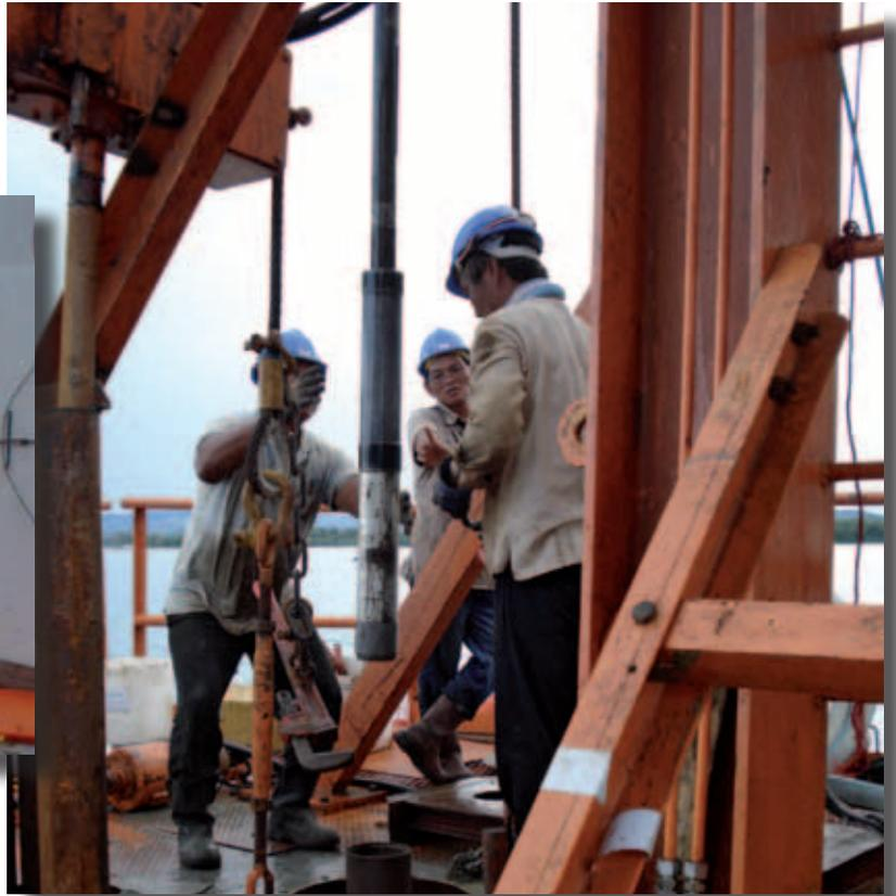
Figure 4. Undertaking undisturbed soil sampling using a ship-mounted rotary drilling rig as part of offshore site investigation works for a major marine development.
