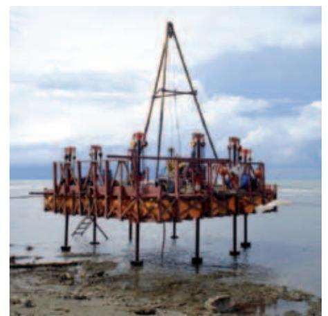
Figure 1. Close-up of the elevated platform for geotechnical sampling through a shallow rock seabed.
