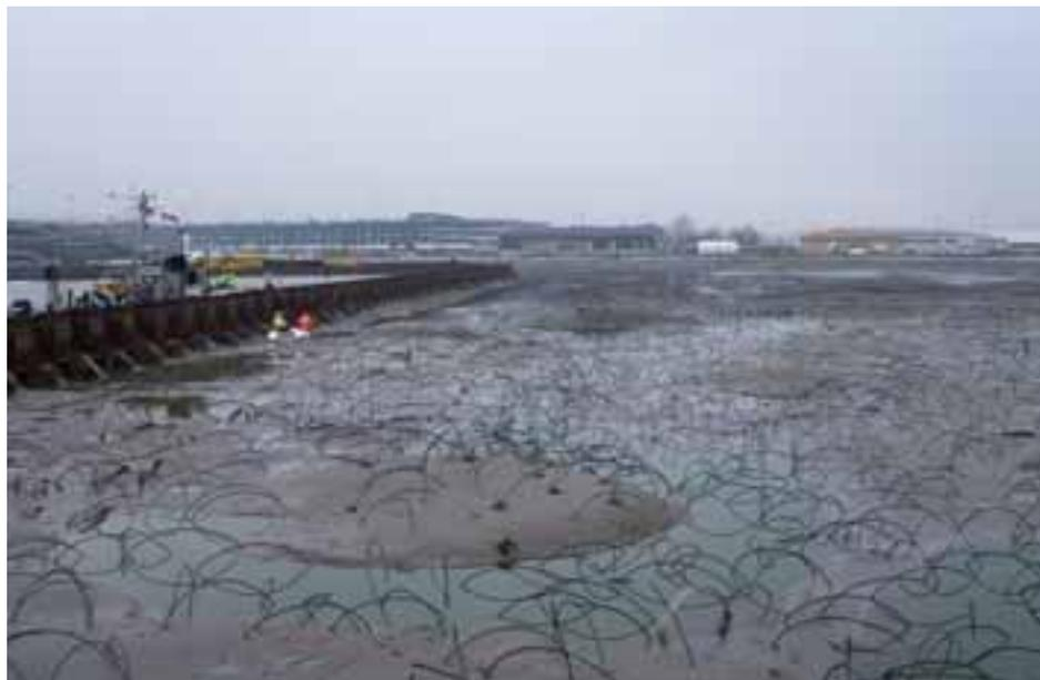
Figure 3. Osthafen depot after the HDPE hoses of the BeauDrain-S system had been pumped dry.
