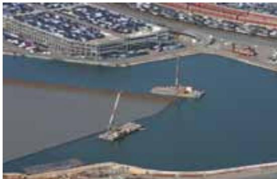
Figure 1. Installation BeauDrain-S from pontoons in the Osthafen depot in Bremerhaven.
