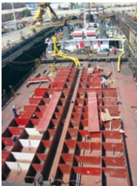
Figure 4. *HAM 602* as she was being converted into a side stone dumper.
