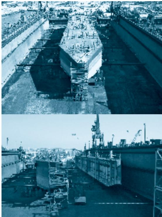
Figure 10. The single pontoon (above) was then separated into two parts (below).
