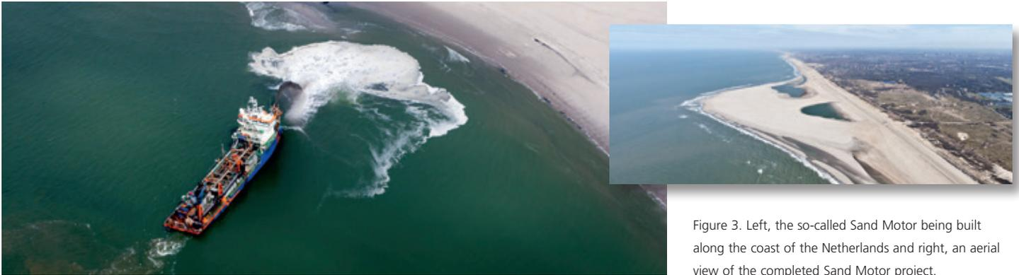
Figure 3. Left, the so-called Sand Motor being built along the coast of the Netherlands and right, an aerial view of the completed Sand Motor project.
