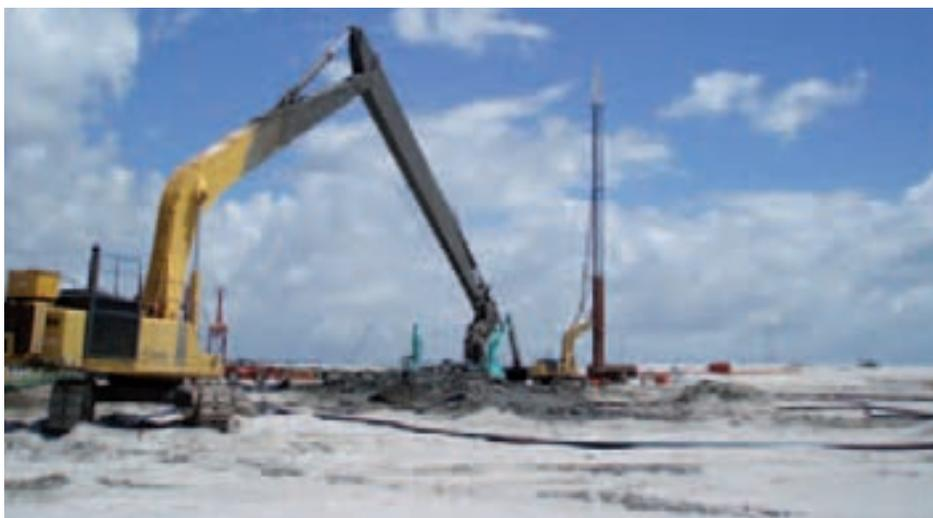
Figure 6. The 80t excavator from Austress Menard excavating the cutoff wall with the PVD installation rig working in the background.
