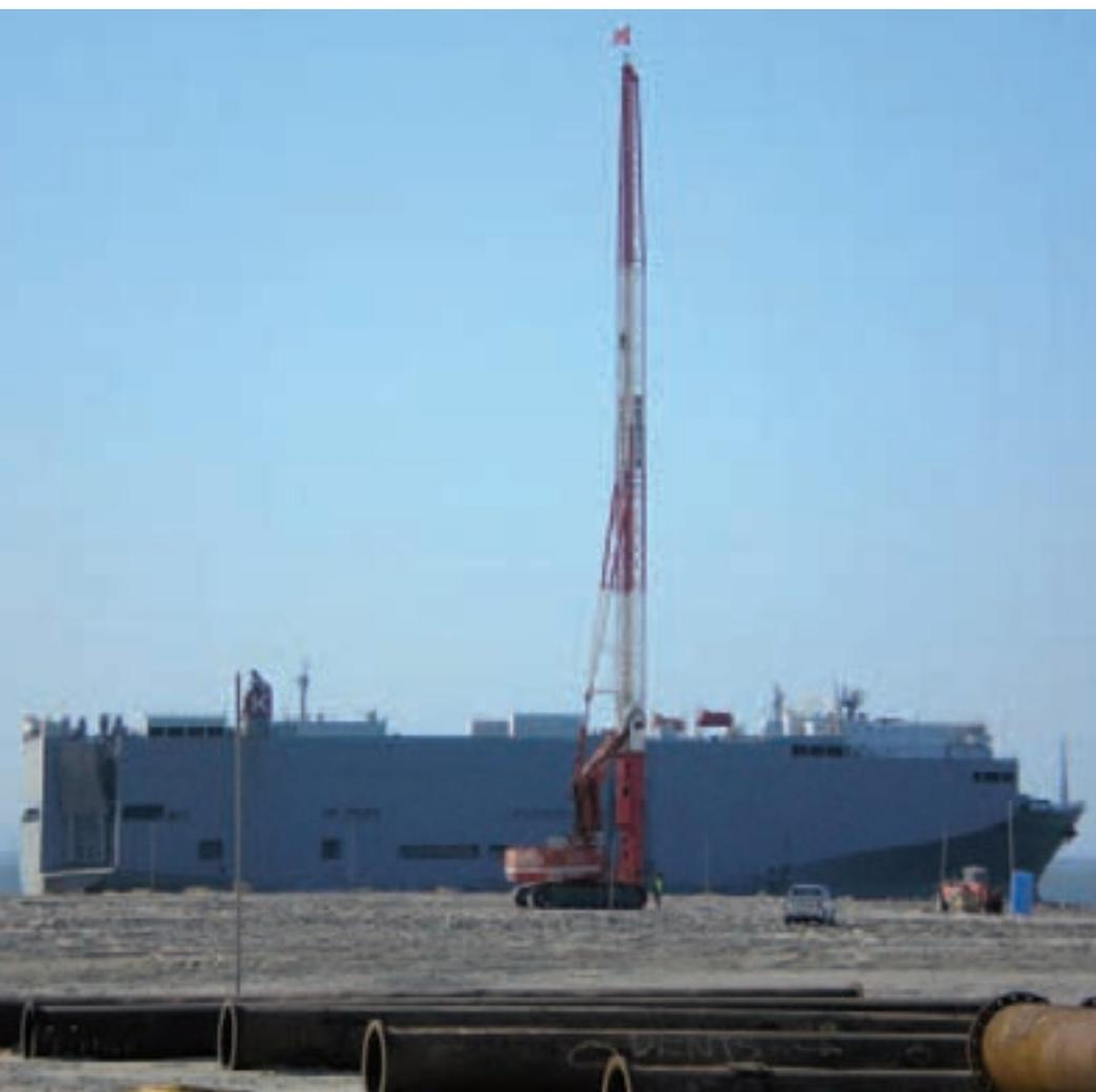
Figure 3. The Boskalis/Cofra rig installing wick drains in the Terminal 11 Trial area. Rig is an 80t machine with 45 metre mast. The dredge pipe is in the foreground. A Car Carrier vessel departing the Brisbane River is visible in the background.
