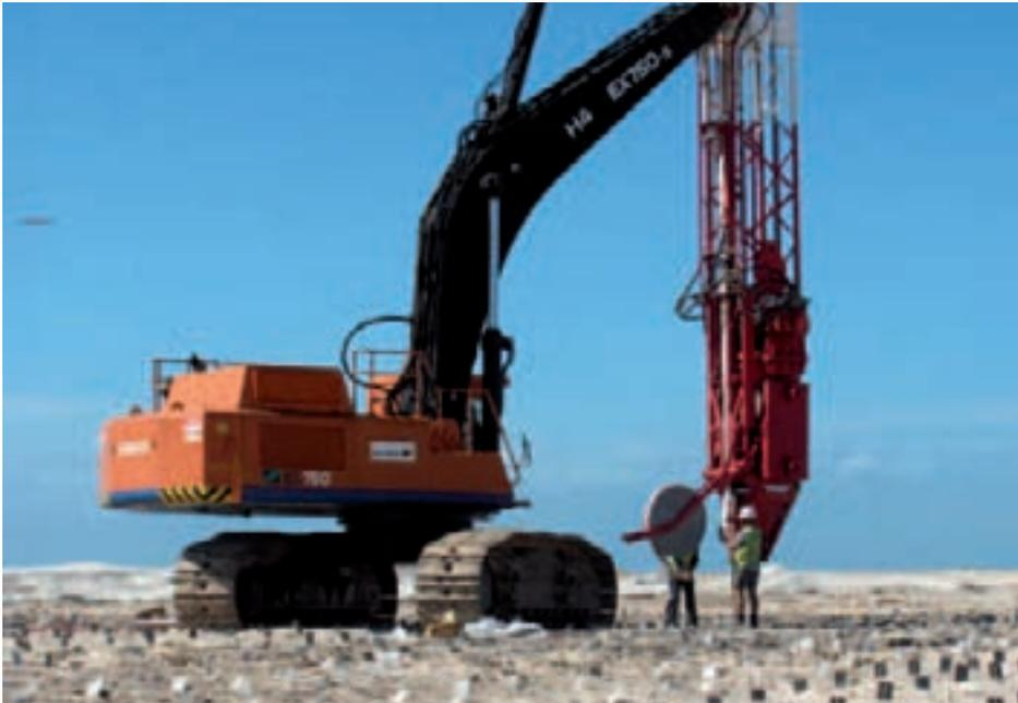
Figure 5. Van Oord is also a trialist in the Terminal 11 Area. Stitching Rig is being filled with new reel of wick drain. Note wick anchor plates used to mark location of each wick prior to installation.
