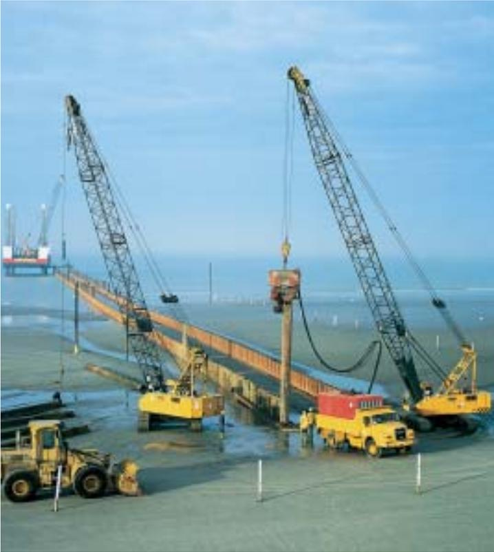
Figure 8. To ensure the safe and stable installation of the pipeline, a 520-m-long and 6-m-wide cofferdam was constructed, partly from the beach outwards and partly from offshore with the aid of a jack-up platform.
