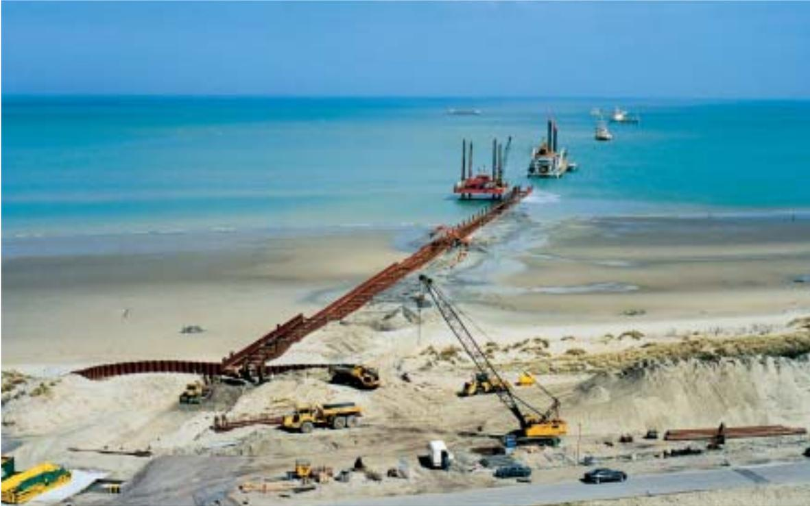
Figure 6. A view from the shore, looking out to sea, of the installation of the cofferdam and winch foundations at Dunkirk.
