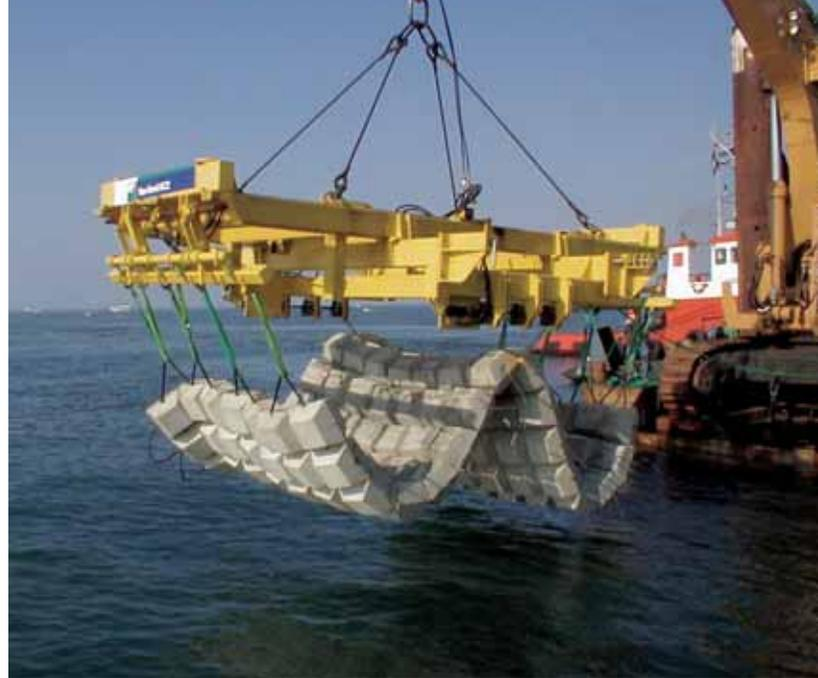
Figure 10. Two views of the installation of flexible concrete mattresses which improved the stability of the pipe. In total 3300 mattresses were installed.
