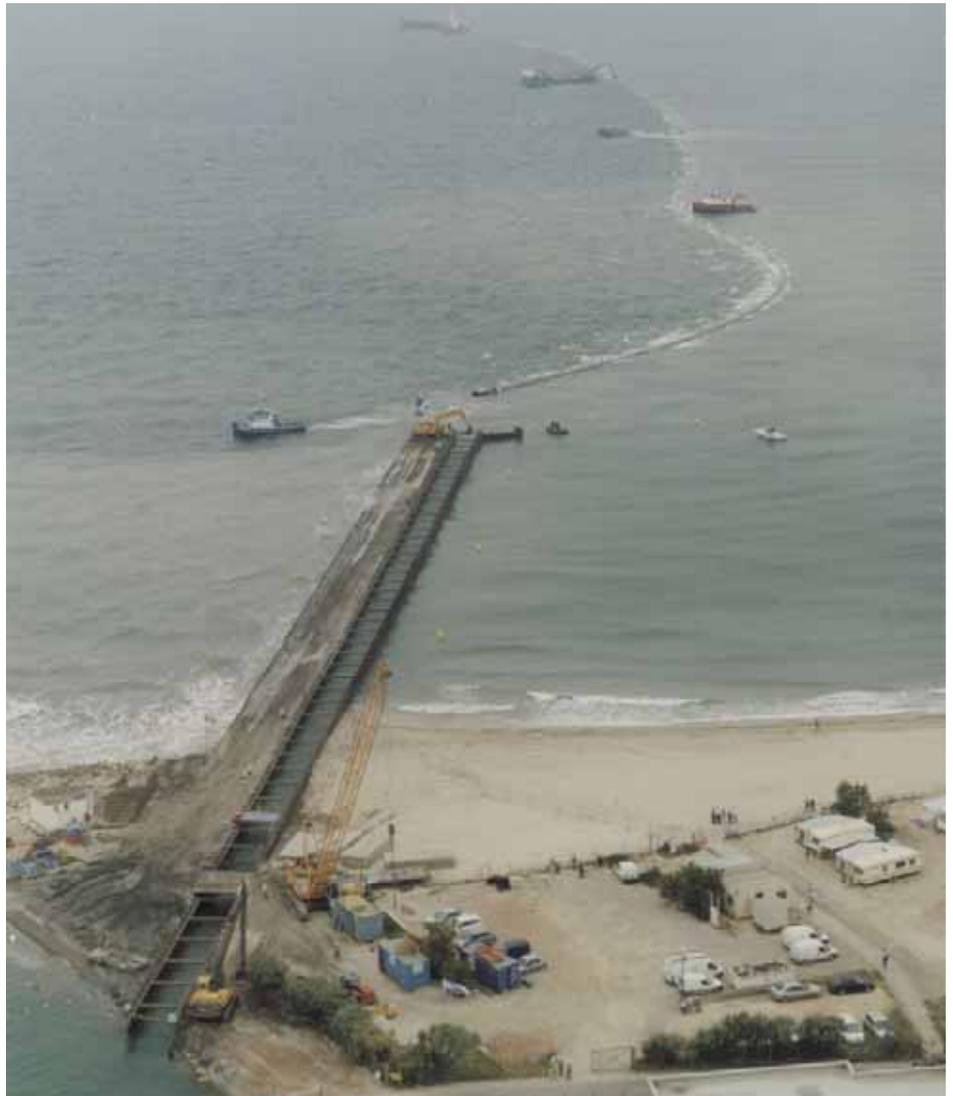
Figure 13. Installation of the first string at site in Palavas.
