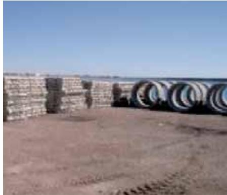
Figure 6. Flexible mattresses and collars stored at construction site in Sète.
