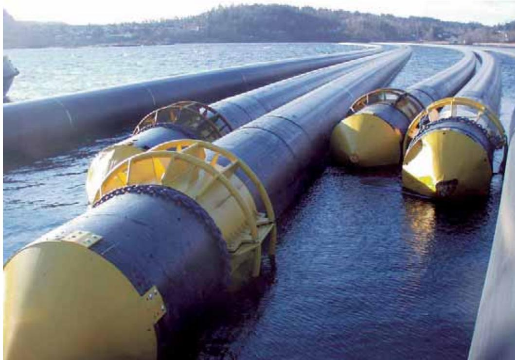
Figure 3. Pipes up to 550 m long were prepared with end plugs and towing clamps for transport by sea.
