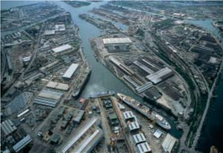
Figure 2. Aerial view of the site of the pilot dredging works in the Northern Industrial Channel of Marghera Harbour.
