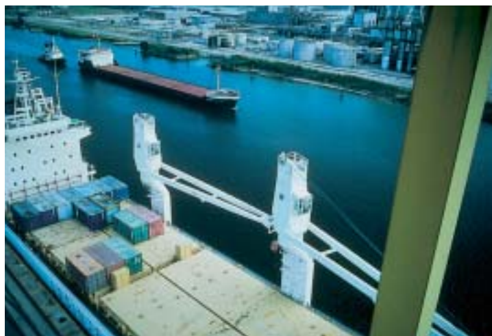
Figure 3. The main navigation channel of Marghera Harbour.
