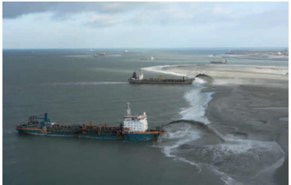
Figure 10. Trailing suction hopper dredgers of the PUMA partners at work on Maasvlakte 2.
