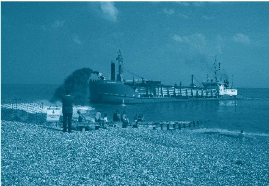
Figure 5. The trailer *Sospan Dau* delivering shingle to the coast.
