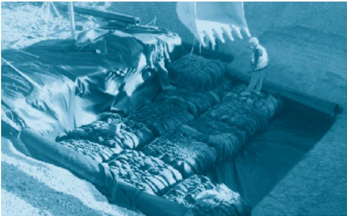
Figure 3. Placement of the bales with car tyres for the coastal defence system.
