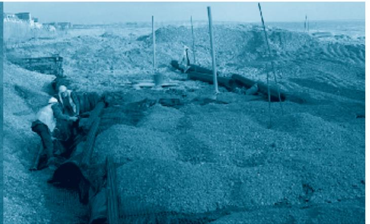
Figure 4. Insulation of the tyre bales.
