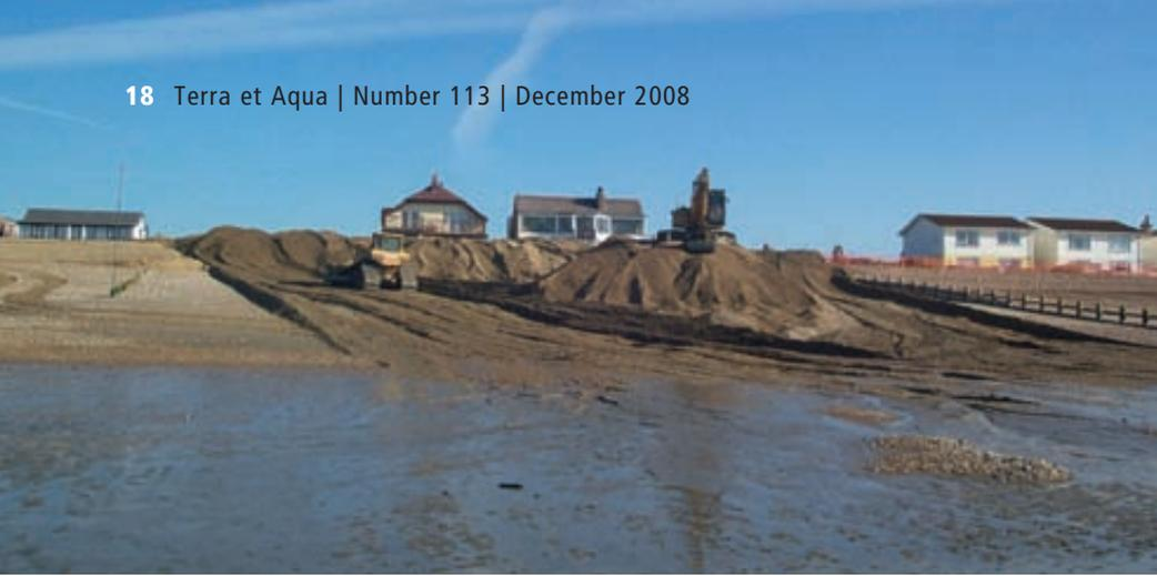
Figure 6. Bulldozers at work spreading the shingle viewed from the sea.
