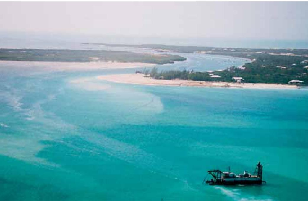
Figure 3. Dredger in operation with beach fill and Leeward-Going-Through in the background.
