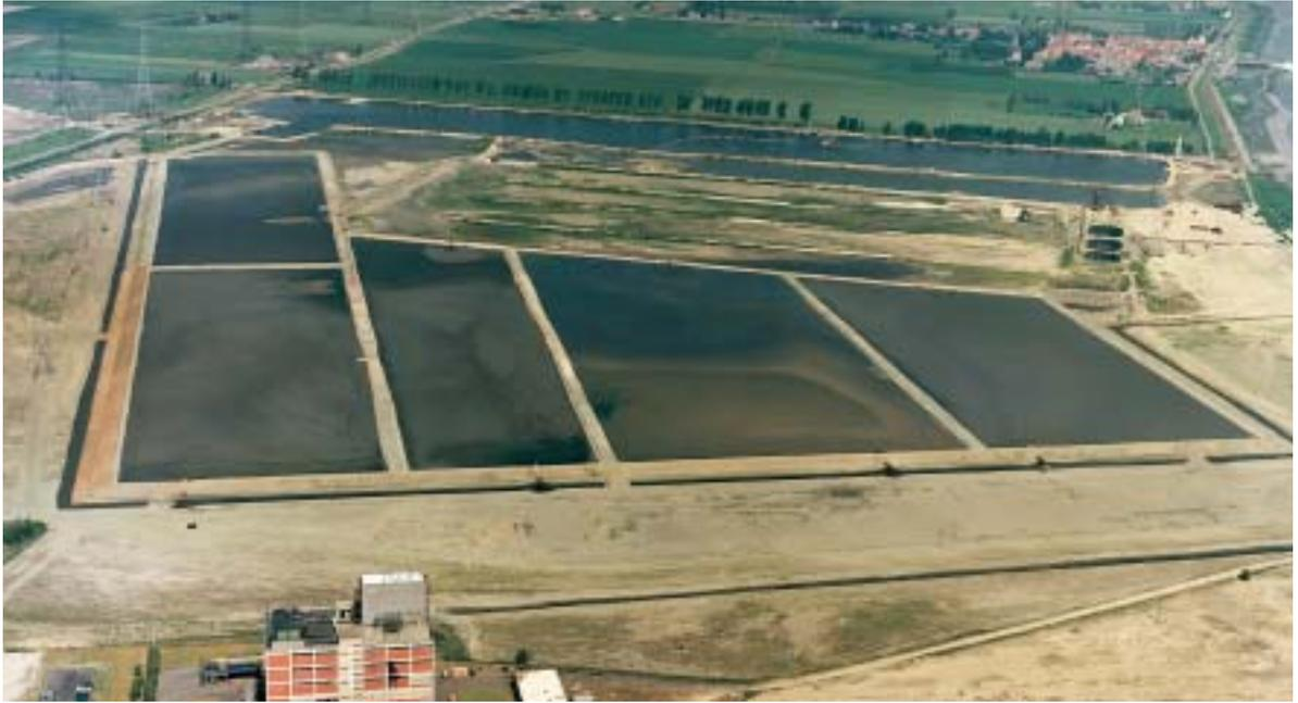
Figure 1. Layout of the dewatering fields.
