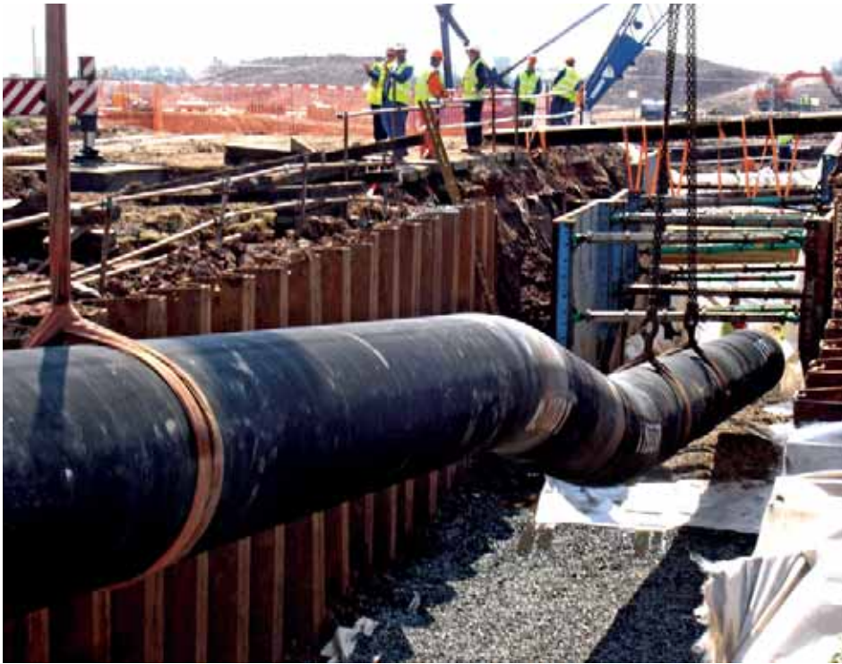
Figure 15. Installation of a spool piece for connection to the main terminal.
