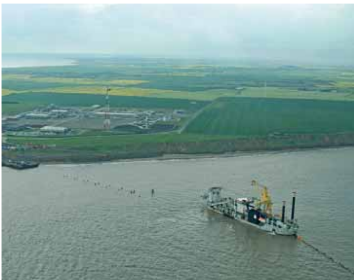
Figure 8. Nearshore trench being dredged by CSD JFJ De Nul.
