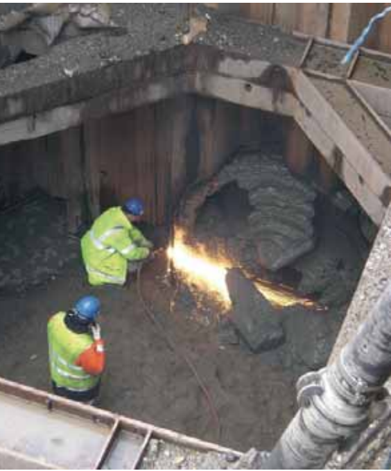
Figure 5. The Tunnel Boring Machine arrives at the tie-in pit.
