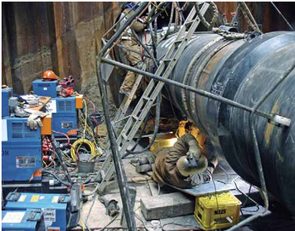
Figure 14. Welding the onshore pipeline.
