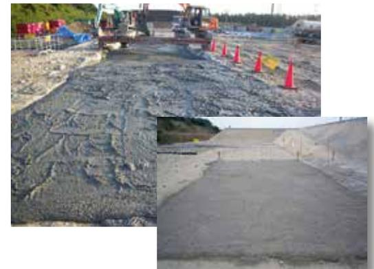
Figure 6. Left, Slag stabilised ground (during placement); and right, slag stabilised ground a year later.
