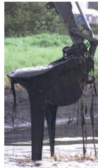
Figure 1. A sample of liquid acid tar as found in the two smaller lagoons. Tar surfaces were covered with a lime slurry specially developed by DEC to prevent emissions of SO<sub>2</sub>.
