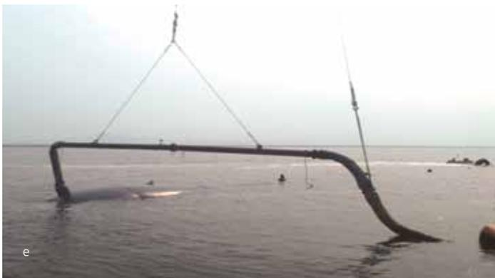
Figure 16. Installation of geotextile tube and formation of sandfill core of the Polder Dike begins with setting out with the GPS equipment and then (a) the laying of basal geotextile (b) laying of geotextile tube (c) attachment of sandbag to weigh down the geotextile tube (d) attaching the filling pipe to the submerged geotextile tube and finally (e) filling of the geotextile tube with dredged sand to design height.
