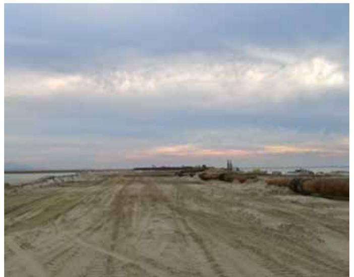
Figure 17. Left, Discharging dredged sand to form sandfill core of the Polder Dike and right, the sandfill core of the Polder Dike surfacing above water level.
