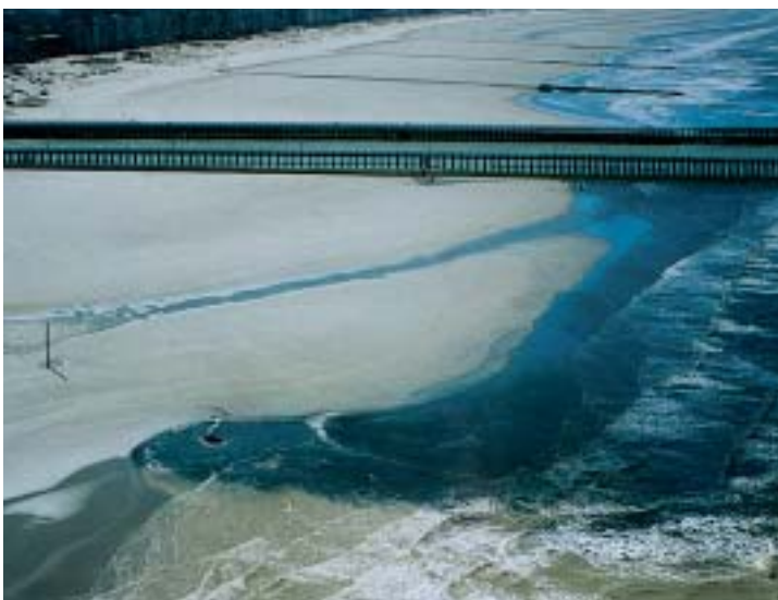
Figure 4. The discharge of the dredged material in the intertidal zone on the beach. The generated plume can clearly be observed.
