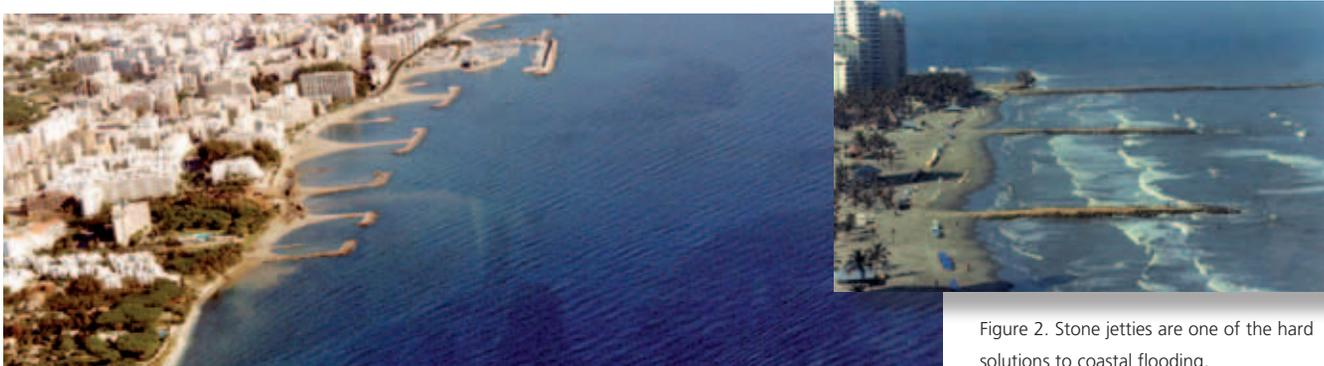
Figure 2. Stone jetties are one of the hard solutions to coastal flooding.
