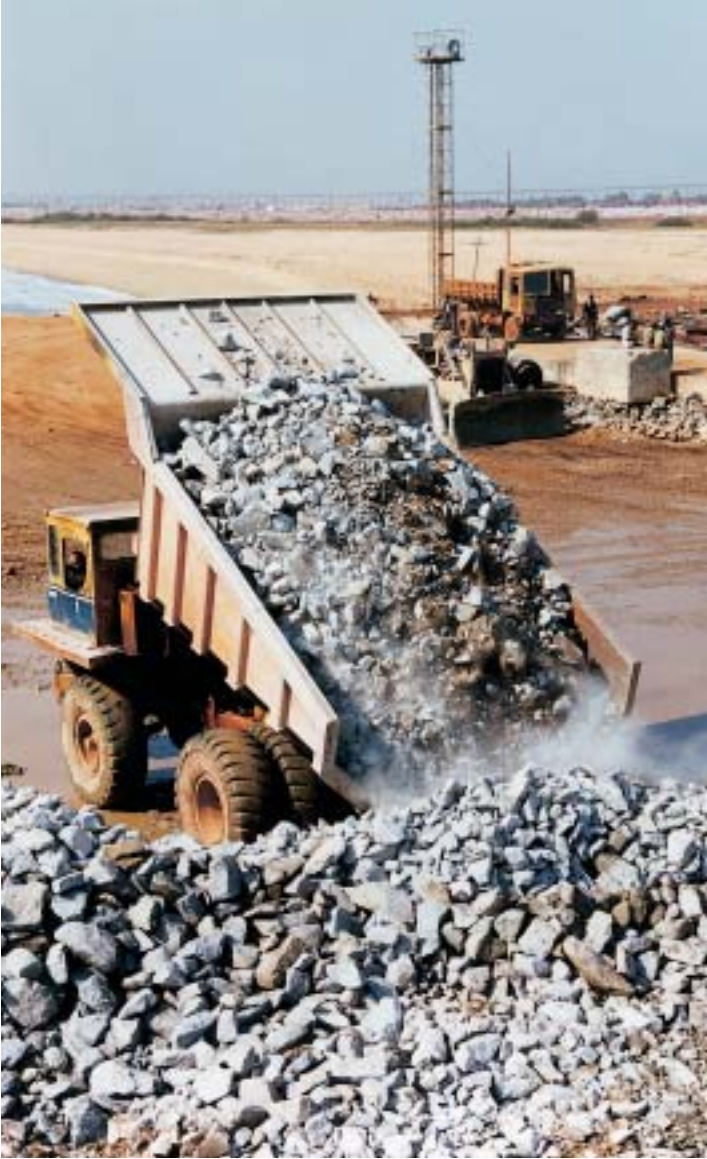
Figure 6. Stone dumpers discharging rock class G at the work harbour.
